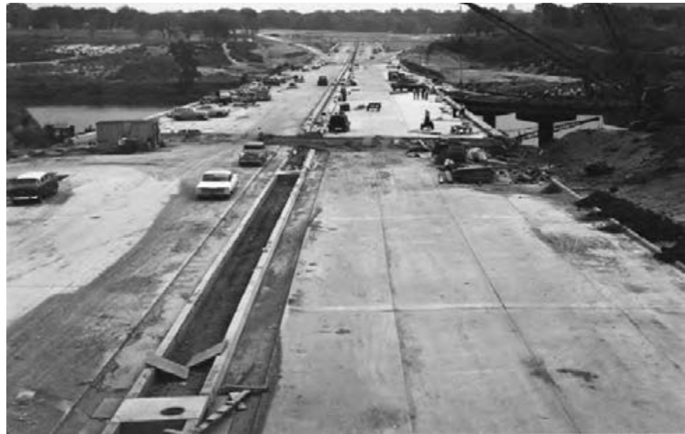
MacVicar Freeway under construction, September 1960. Walter Van Horne Collection, State Historical Society of Iowa, Des Moines.
