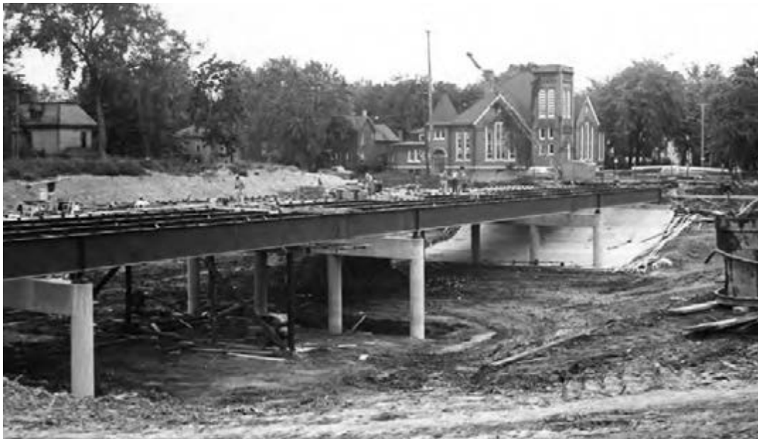
MacVicar Freeway overpass under construction, September 1960. Walter Van Horne Collection, State Historical Society of Iowa, Des Moines.
